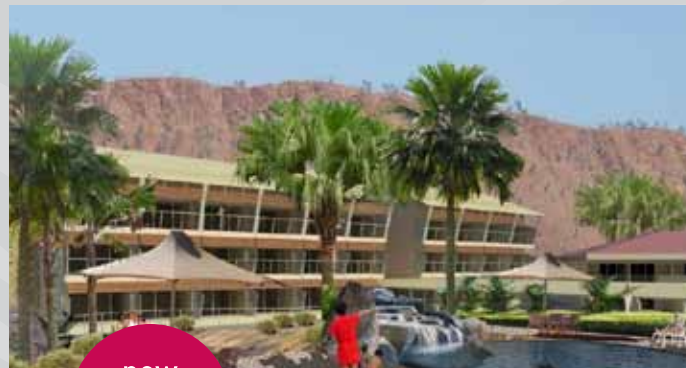
new hotel block and pool
